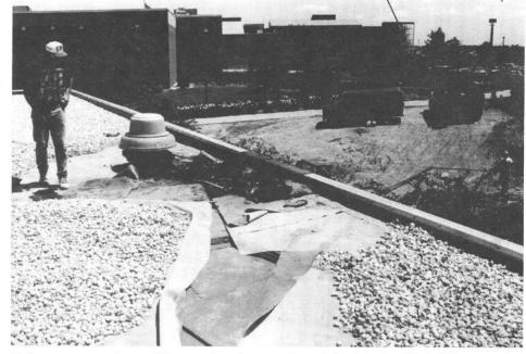
College personnel are still assessing damage from lightning that hit Building U on Sunday, July 18. Lightning struck the roof exhaust fan of the Ceramic Studio, and rain damaged the kiln below. Computers in an adjacent building also malfunctioned after the incident.
