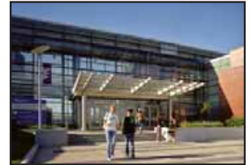
The Avanté Center houses state-of-the-art information technology equipment.
