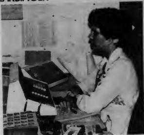
Photo by Neil Hingorani Penny Jaskey at the main switchboard of Harper College. The new boards have been in use since July 25.
