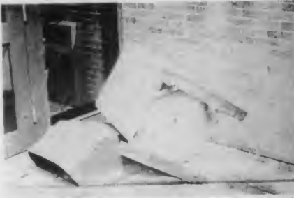
A BROKEN WINDOW in D building and one of several overturned garbage cans was part of the rubble left after last Friday's disturbance. Photo by Kathy Kowalik.
