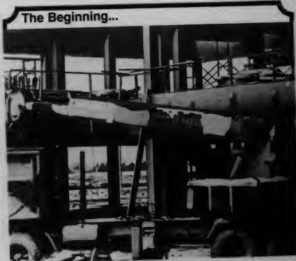
Ground was broken in 1967 for Harper College and students and faculty anxiously awaited completion of buildings. Prior to the permanent Palatine campus being established, classes were held at Elk Grove and Forest View High schools.
