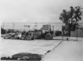
Tennis courts get needed renovation.
