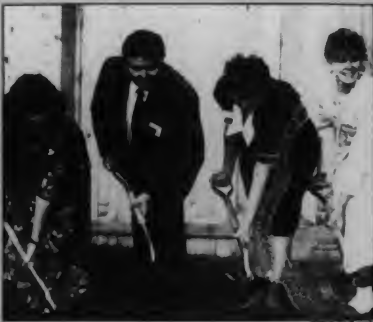
Harper College President James T. Wrenson, center, will officiate at the ground breaking for the new 'L' building.
