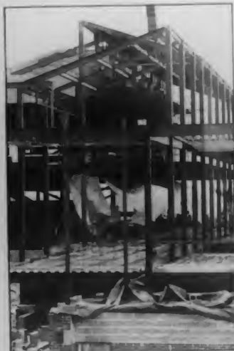
BUILDING I will be home of the new Block Box
