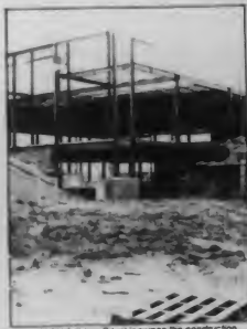
VIEW FROM Building C looking upon the construction
