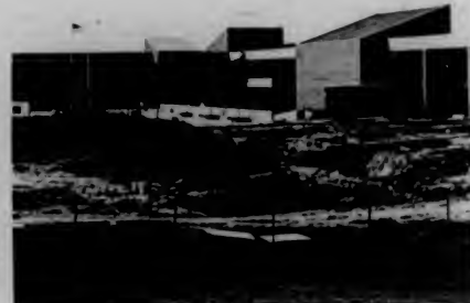
Two views of the site of the new music wing.
